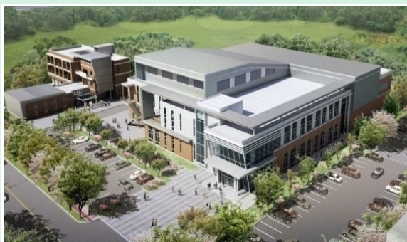
Bird's-eye view of the Ultrashort Quantum Beam Facility
