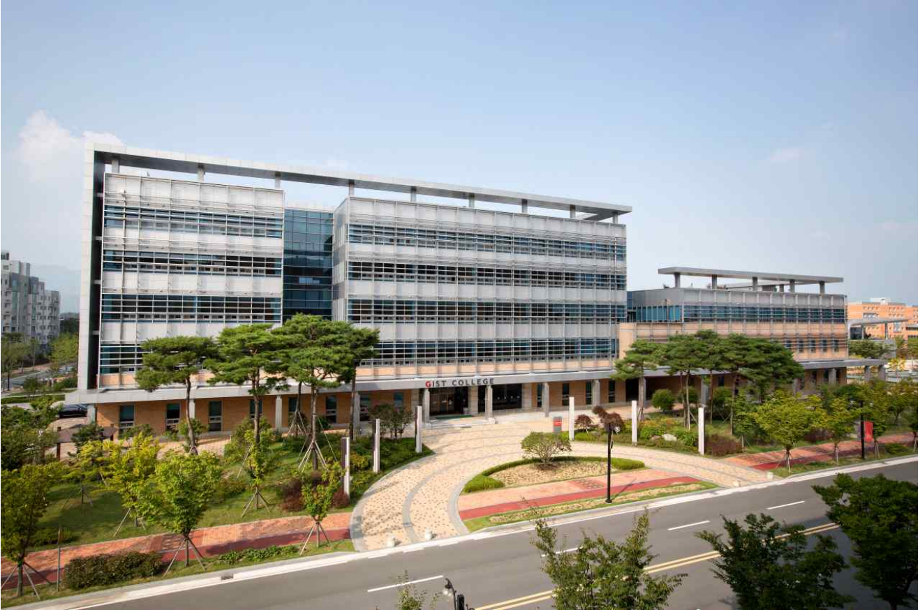
▲ Photo: GIST College Building A
