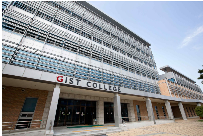
▲ Photo 1. GIST College Building A
