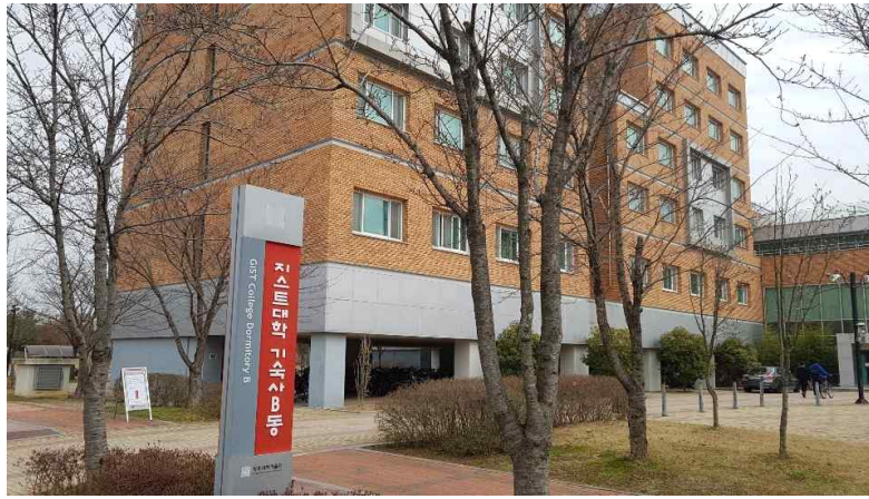
(Photo 1) College dormitory building used as the COVID-19 isolation building
